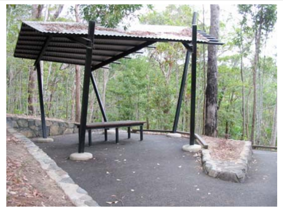
Second shelter shed
