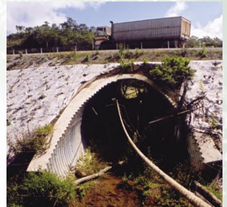
An operational underpass shortly after completion of the East Evelyn upgrade, on the Atherton Tablelands (Image: Jonathon Munro).
