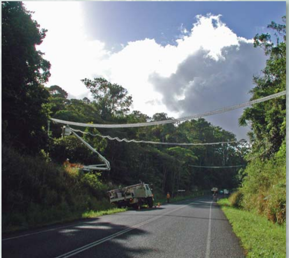
New rope bridges for tree-dwelling animals were erected in November 2005 across the Palmerston Highway between Innisfail and Millaa Millaa in a collaborative effort by the Rainforest CRC, Queensland Department of Main Roads, Environment North and Ergon Energy (Image: Birgit Kuehn).
