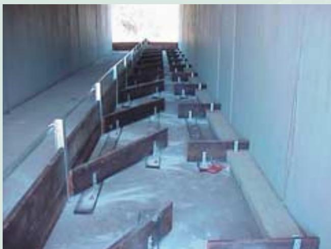
LOOKING UPSTREAM: University Creek prototype culvert fishway
