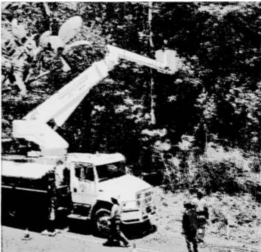
Poles apart: An Ergon Energy cherry picker crew hangs the start of a rope bridge over the Palmerston Highway, west of Innisfail, to allow canopy dwellers to cross the busy road in safety.
