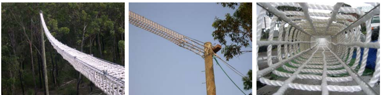
Figure 3. Close up views of a typical rope crossing.
