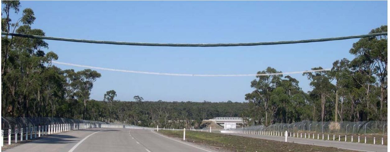
Figure 4. Two of the rope crossings, one closed with headlight glare protection
