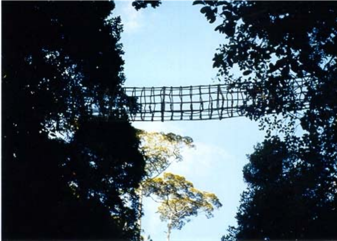
Figure 6.1. Study site. The existing canopy bridge was erected by Department of Environment personnel (Rupert Russell) on the B road (Kauri Creek Road) in the Lamb Range road network using funding provided by the Wet Tropics Management Authority.
