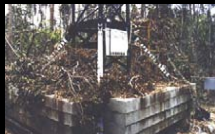
Damage caused by Category 3 tropical cyclone Rona.
