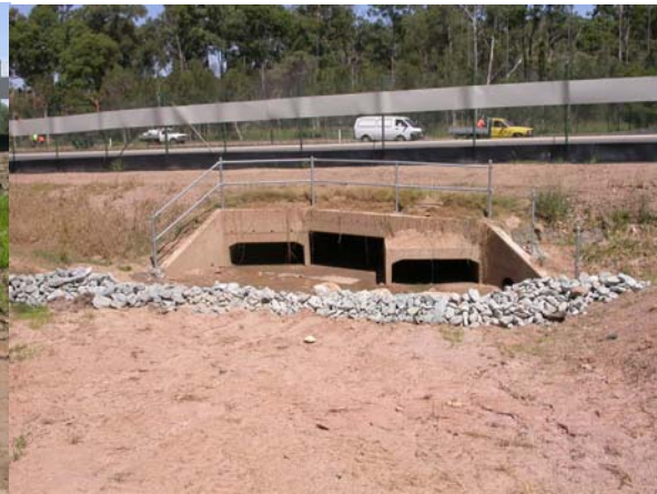
Figure 9. Three-box wet culvert. (Photo: Pauline Fitzgibbon)
