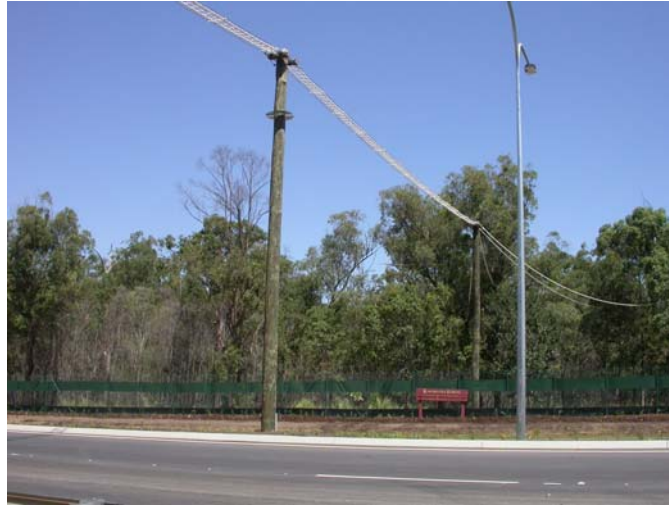
Figure 20. Rope bridge as currently constructed at Compton Road (Photo: Pauline Fitzgibbon). It is strongly recommended that the 4 ropes connecting the trees with the pole on which the rope bridge is mounted at either end of the bridge be converted to lengths of rope bridge as the bridge structure should be actually touching the trees to encourage animals to use it.
