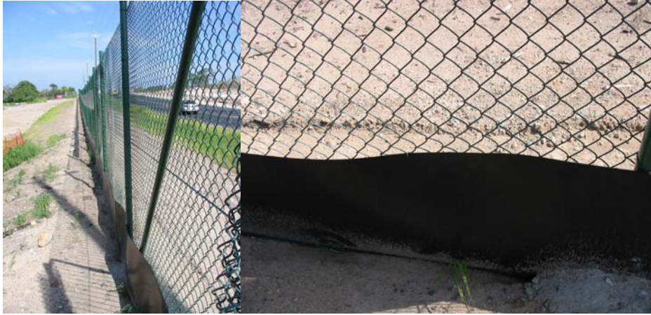
Figure 7. Fauna exclusion fencing with mesh above to deter large species and solid plastic barrier buried into the soil to deter small mammals, amphibians, lizards and snakes.
