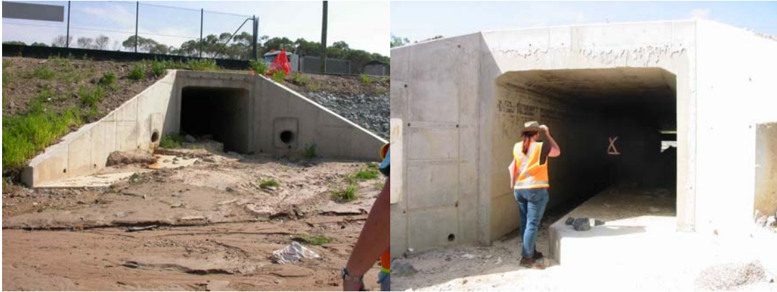
Figure 4. Modified box culverts with ledge to allow dry passage for fauna during low rainfall events.
