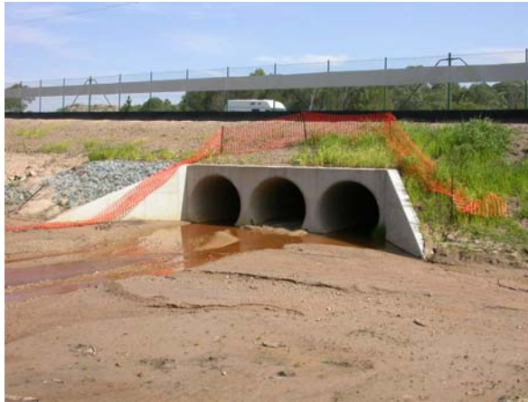
Figure 8. Three-pipe wet culvert. (Photo: Pauline Fitzgibbon)
