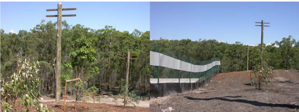
Figure 6. Glider poles situated on top of land bridge (Photos: Pauline Fitzgibbon).
