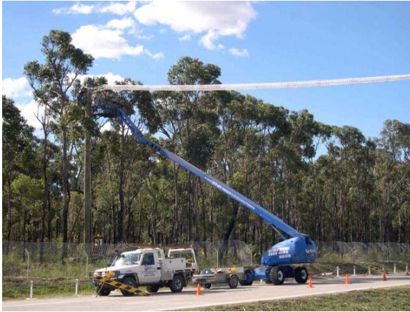
Figure 21. Rope tunnel erected in New South Wales.
