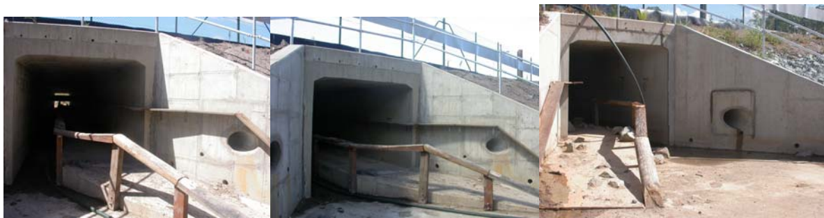
Figure 17. Faunal underpasses with faunal furniture installed at Compton Road.
